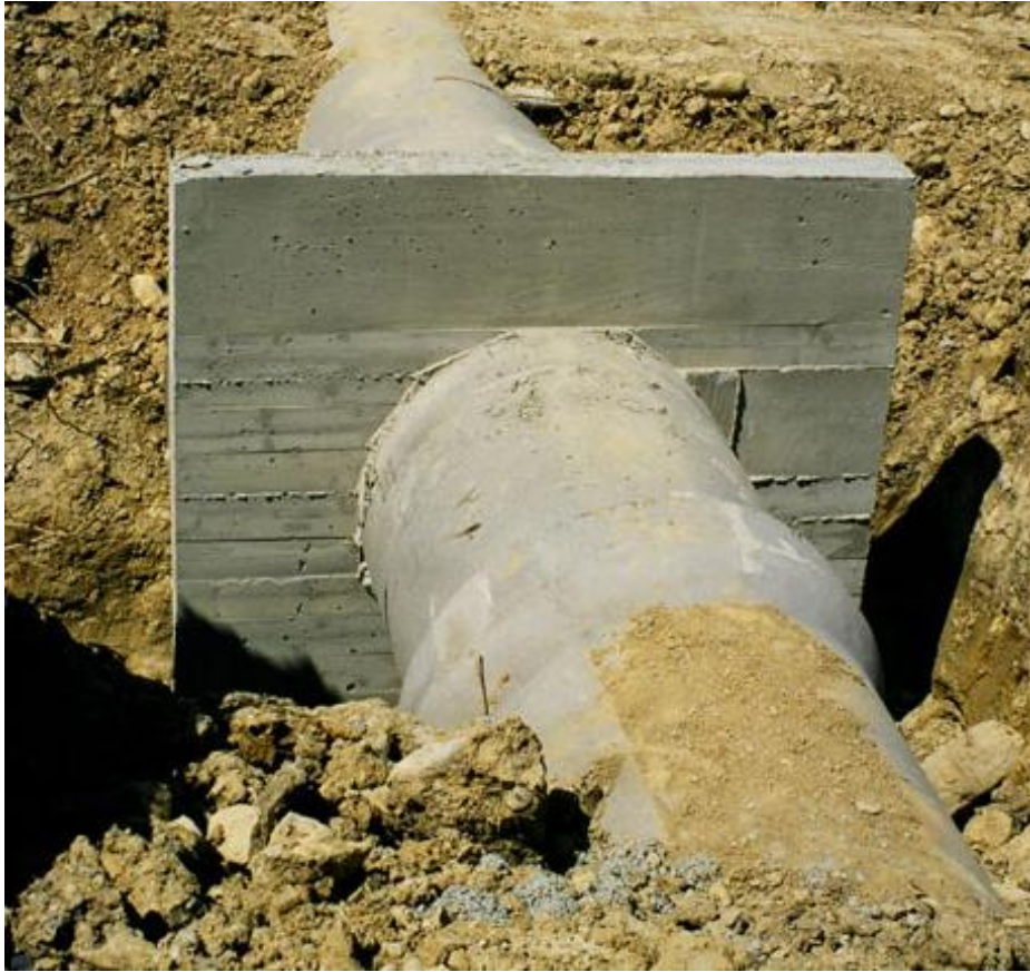
FIGURE 7.6 Anti-seep Collar Design
