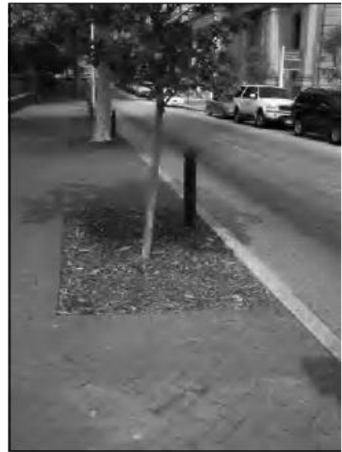
Although 5 by 5 by 3 feet to 6 by 6 by 3 feet are the recommended minimum cutouts, larger planters such as 6 by 12 by 3 feet should be used to plant large trees in downtown areas.
